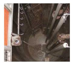
into the wastewater stream. The facility's "non-clog" submersible pumps, installed in a 20-foot-deep wet well, couldn't handle the plastic
